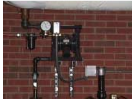
Figure 20: Engine Crankcase Oil Pump for oil changes
