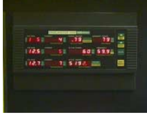
Figure 4: Single Waukesha engine data screen
