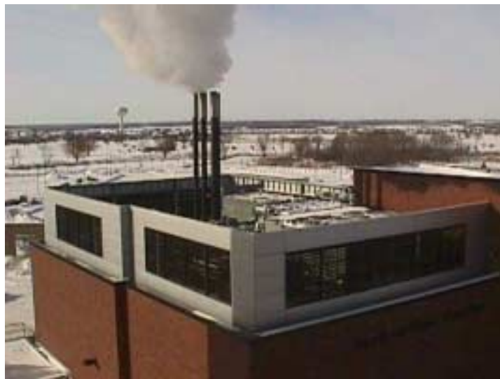
Figure 2: ECC's Cogenerating Plant
