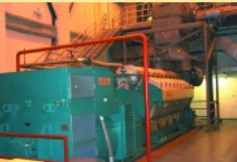
Newly installed 3.8-MW Wärtsilä engine-generator in the central plant at UIC. These lean-burn engines are characterized by high electrical efficiency, dependable operation, and low maintenance costs.
