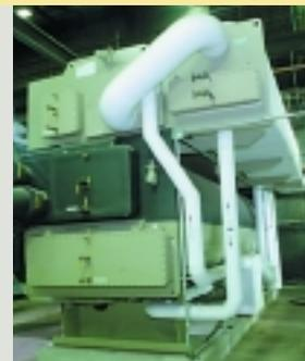
New 1,000RT Trane Double Effect Absorber high-temperature hot-water-activated water chiller
